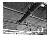
If you see a pipe leaking in the garage, please note what color it is when reporting it. Water and sewer drain lines are white in color. The blue and green striped pipes are water loop lines that service the cooling tower/HVAC system.
