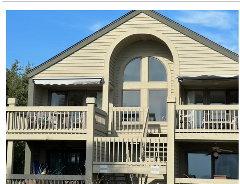
Figure 3c Entrance Outside Corner Window
