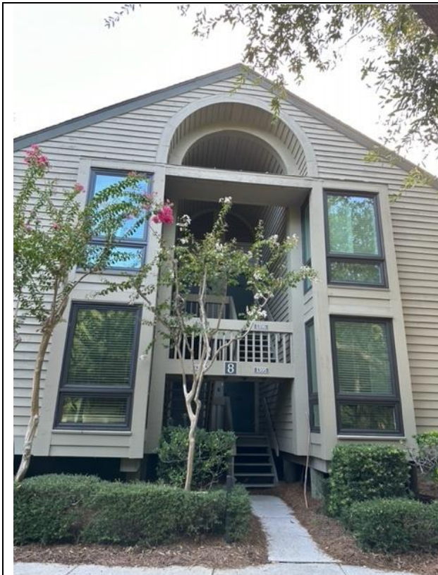
Figure 3b-1 Entrance Front Window
