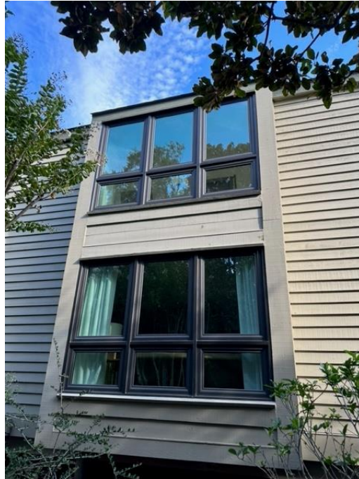
Figure 3b-3 Entrance Outside Corner Window
