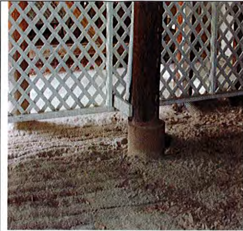
Figure 1 Piling encapsulation repair
