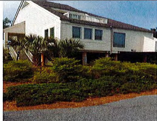
Figure 25 Lower Level Porch Enclosure
