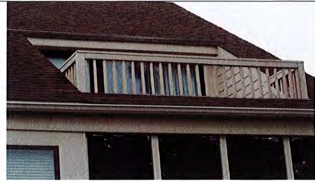
Figure 30 Upper level deck with railing
