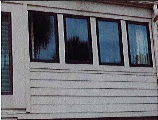
Figure 24 Lower Level Porch Enclosure
